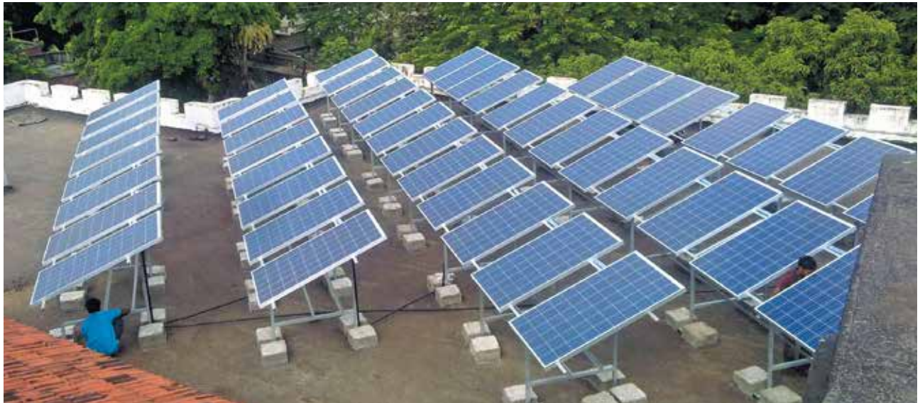
Roof Top Structure
