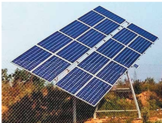
Single Axis Structure
