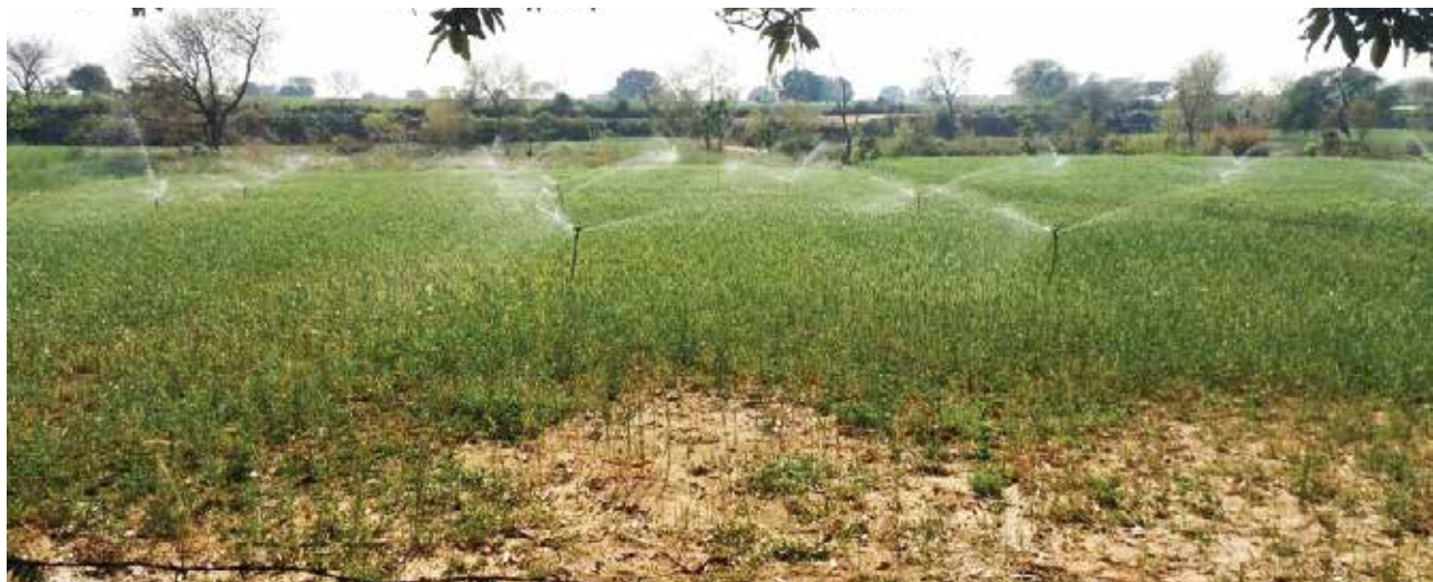
Jain Solar Pumping Station for Integrated Micro Irrigation Project, Talwara, Punjab
