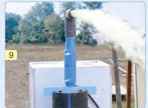
9 The well is ready to use
