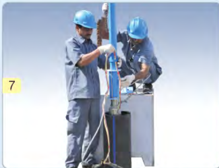
7 Lock the Cable using Cable Clip
