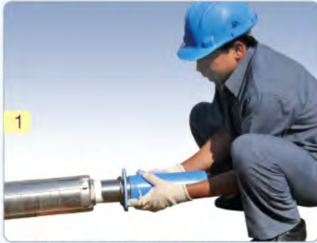
1 Connect the Pump Connector with the Pump
