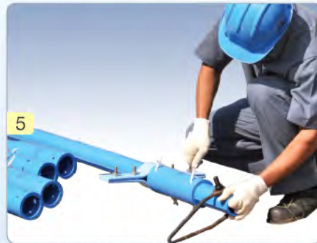
5 Prepare the Pipe for Lowering
