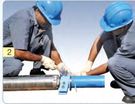
2 Mount the Holding Clamp
