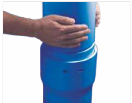
Push the spigot into the socket
