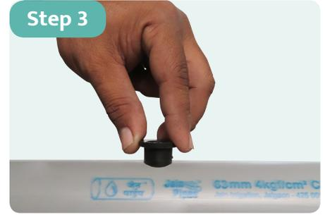
Insert the Top Hat Grommet fully. Ensure that the collar is resting on the pipe wall.
